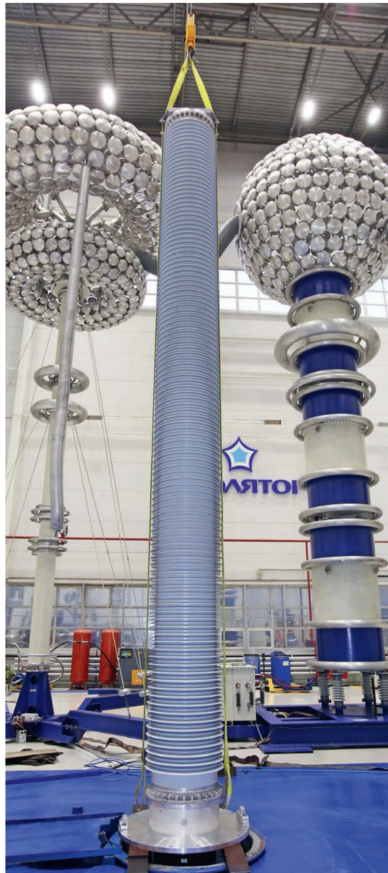
Installation of the bushing on the test tank for acceptance testing
