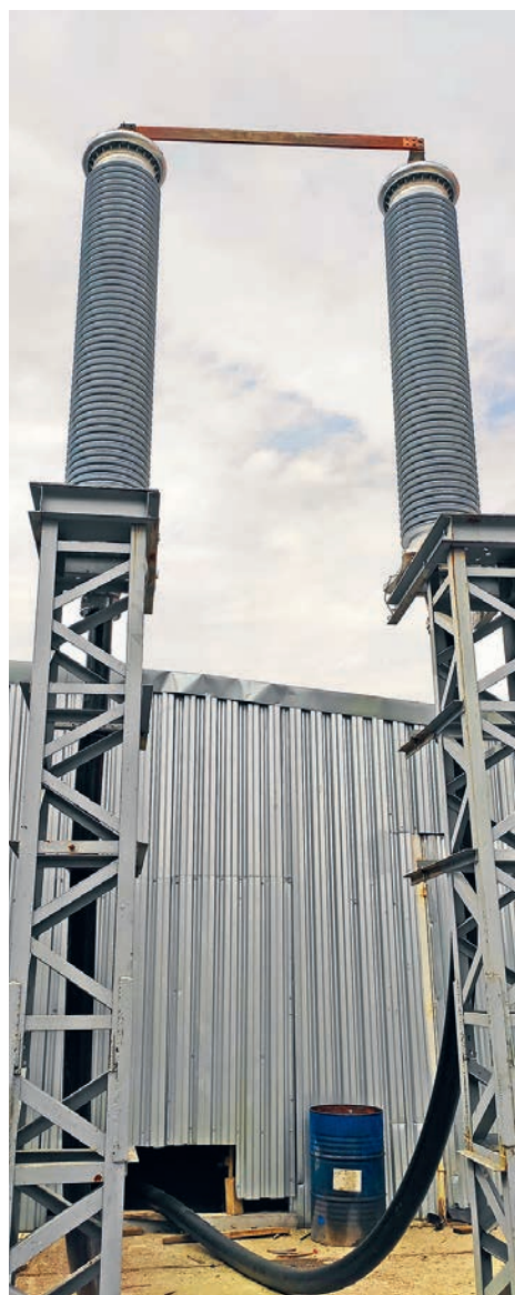
Pre-qualification tests of Izolyator-AKS IKM-252 cable terminations in the testing center of the Russian Cable Scientific Research and Development Institute
