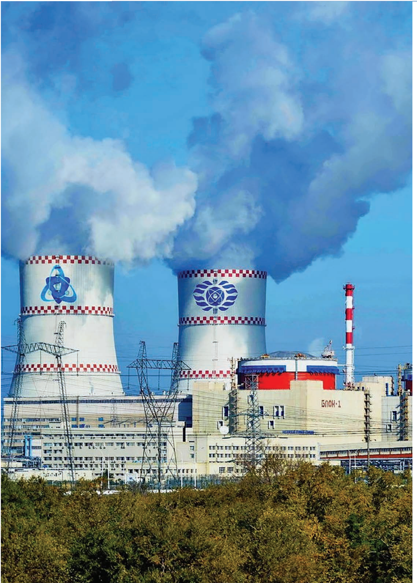
Rostovskaya NPP of Rosenergoatom — partner of Izolyator Group
