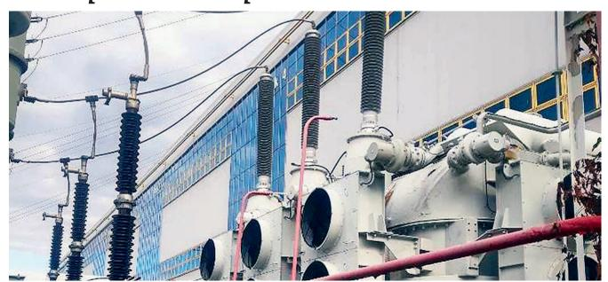
240 MVA transformer with 252 kV Izolyator bushings at Dolna Odra power plant in Poland
