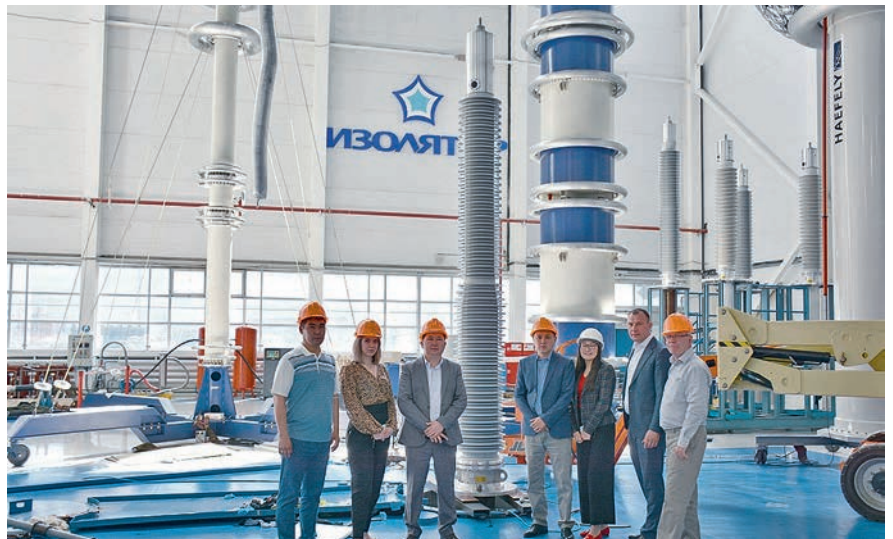
Representatives of the National Electric Grid of Kyrgyzstan during the inspection of Izolyator high-voltage bushings. In the background – a 500 kV bushing under test
