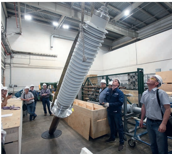
Practicing the operation of setting the bushing into a vertical position after removing it from the packaging
