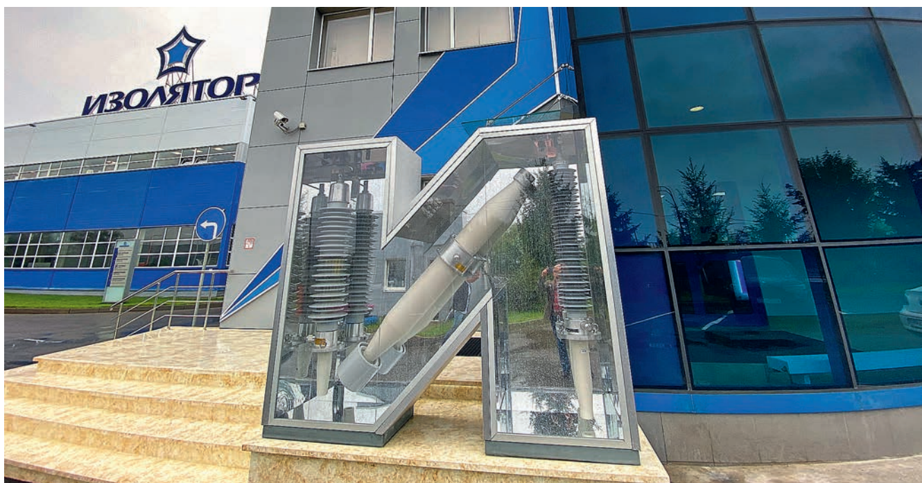
The renovated entrance group of the administrative wing of Izolyator complex
