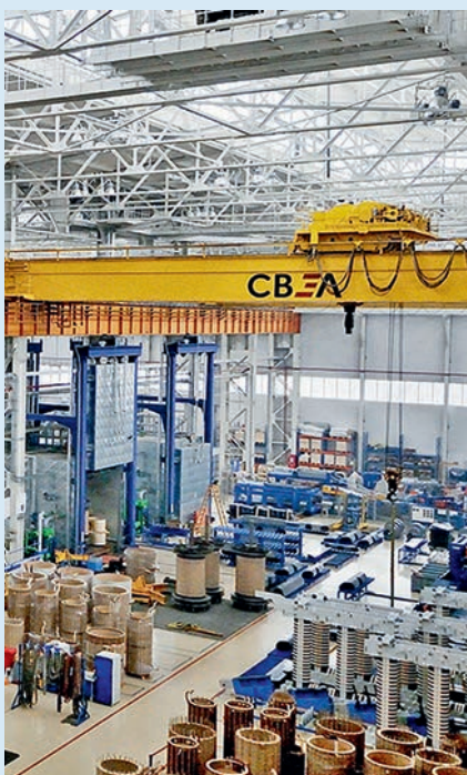
SVEL - Power Transformers plant (photo: SVEL Group)
