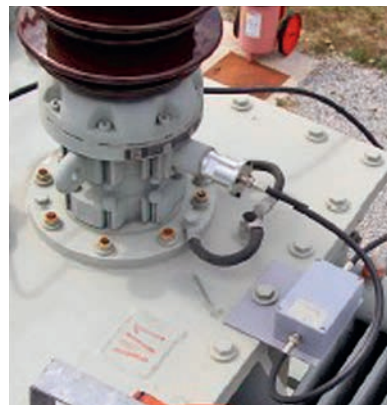
Fig. 1 Connecting to the measuring tap
