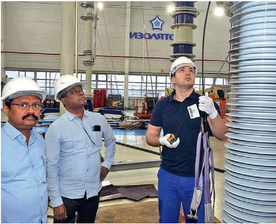
Inspection of HV bushings tests by specialists of the state power grid company of the Indian state Telangana Transmission Corporation of Telangana Limited (TSTRANSCO)
