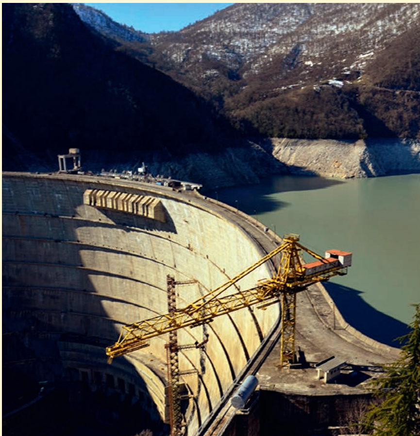
Inguri Hydroelectric Power Plant (Photo: Chernomorenergo RUE)
