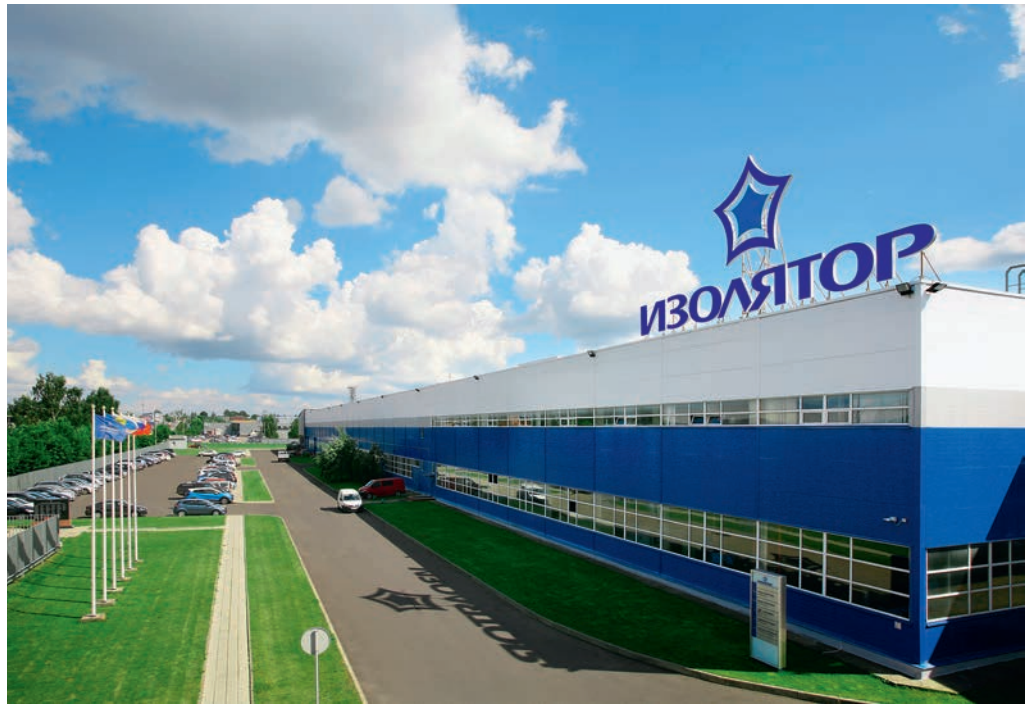
Production facility of Izolyator
