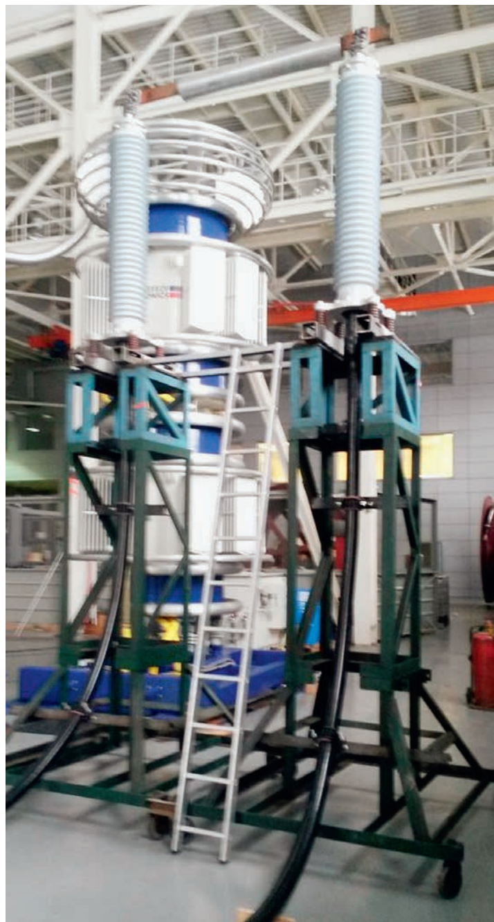
End sleeve fitting at the test laboratory
