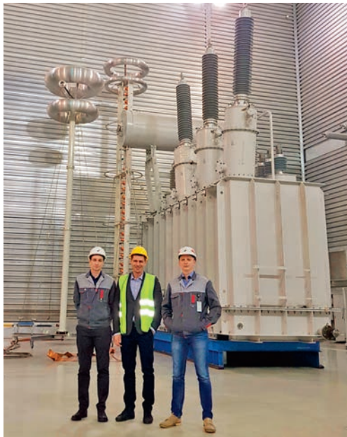
At the Power Machines - Toshiba High-voltage Transformers plant, L-R: PMTT Business Development Director Konstantin Stafeev, Maxim Zagrebin, and PMTT Senior Design Engineer Alexander Smimov. In the background to the right - a transformer with 252kV high-voltage bushing produced by Izolyator.
