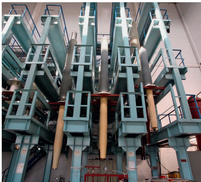
RIN bushings on manufacturing racks at the assembly shop of Izolyator
