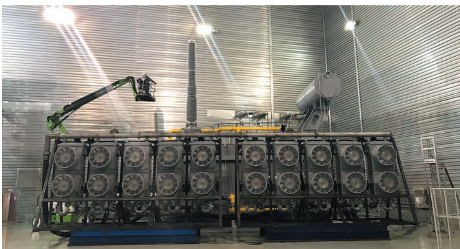
A 750 kV Izolyator RIP bushing installation on a PMTT transformer intended for Kalinin NPP
