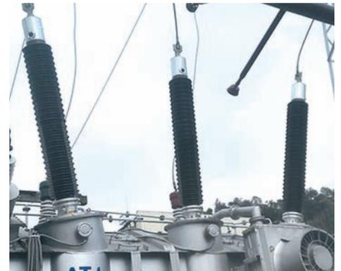
220 kV transformer RIP bushings made by Izolyator, installed in 2016
