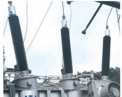
220 kV transformer RIP bushings made by Izolyator, installed in 2016
