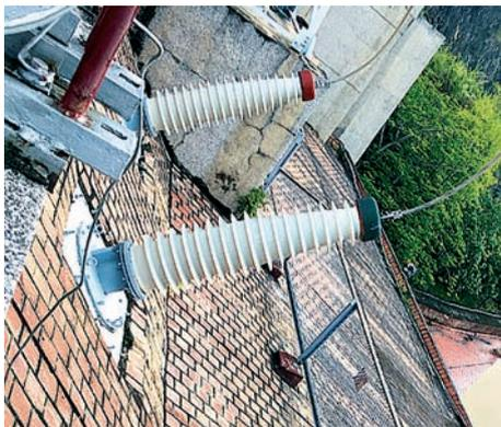
220 kV wall bushings made by Izolyator in operation for over 25 years
