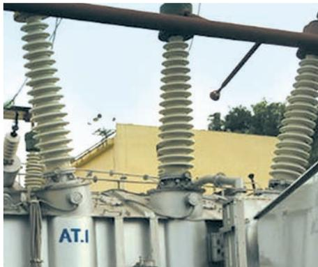
220 kV OIP transformer bushings made by Izolyator with over 25 years operation period
