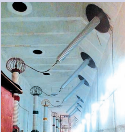
Installation of 220 kV RIP bushings from the first lot of Izolyator's wall bushings received at Hoa Binh HPC in 2017
