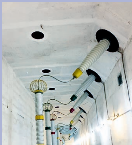
220 kV OIP wall bushings have operated for over 30 years at Hoa Binh HPC
