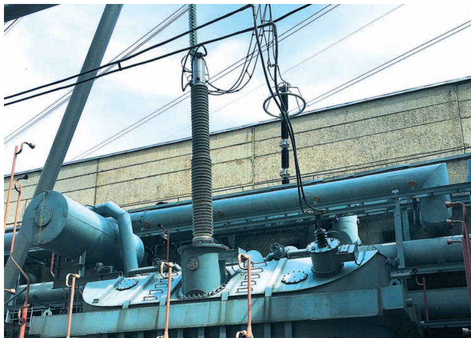
500 kV Izolyator RIP bushing in a block transformer at Krasnoyarskaya HPP
