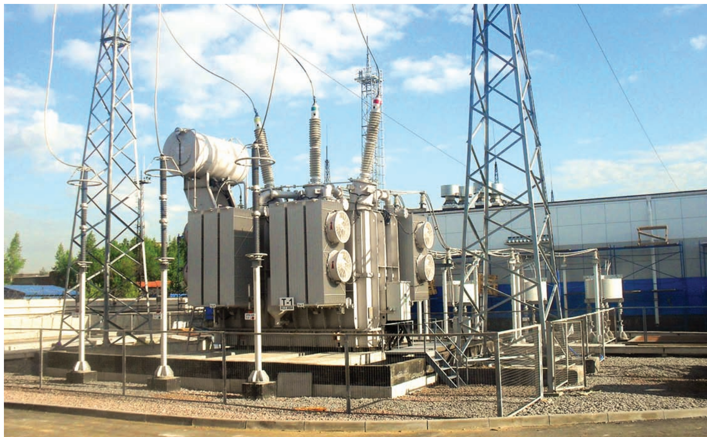
220 kV Izolyator bushings in a transformer of MES North West (photo courtesy FGC UES)
