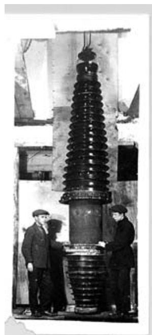
Exterior appearance of a bushing with oil-barrier insulation
