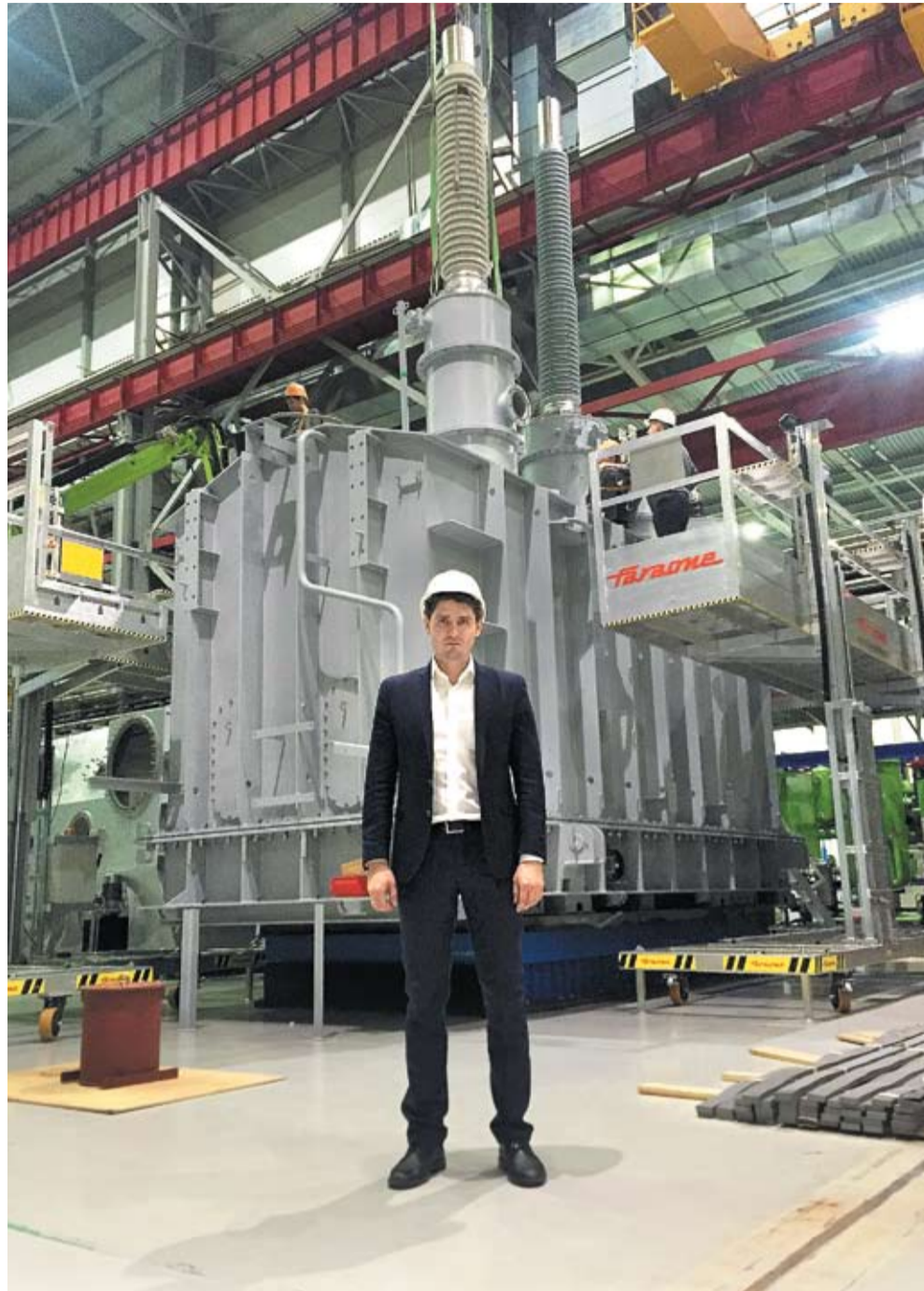
Maxim Zagrebina at Power Machines – Toshiba. High-voltage transformers Ltd plant
