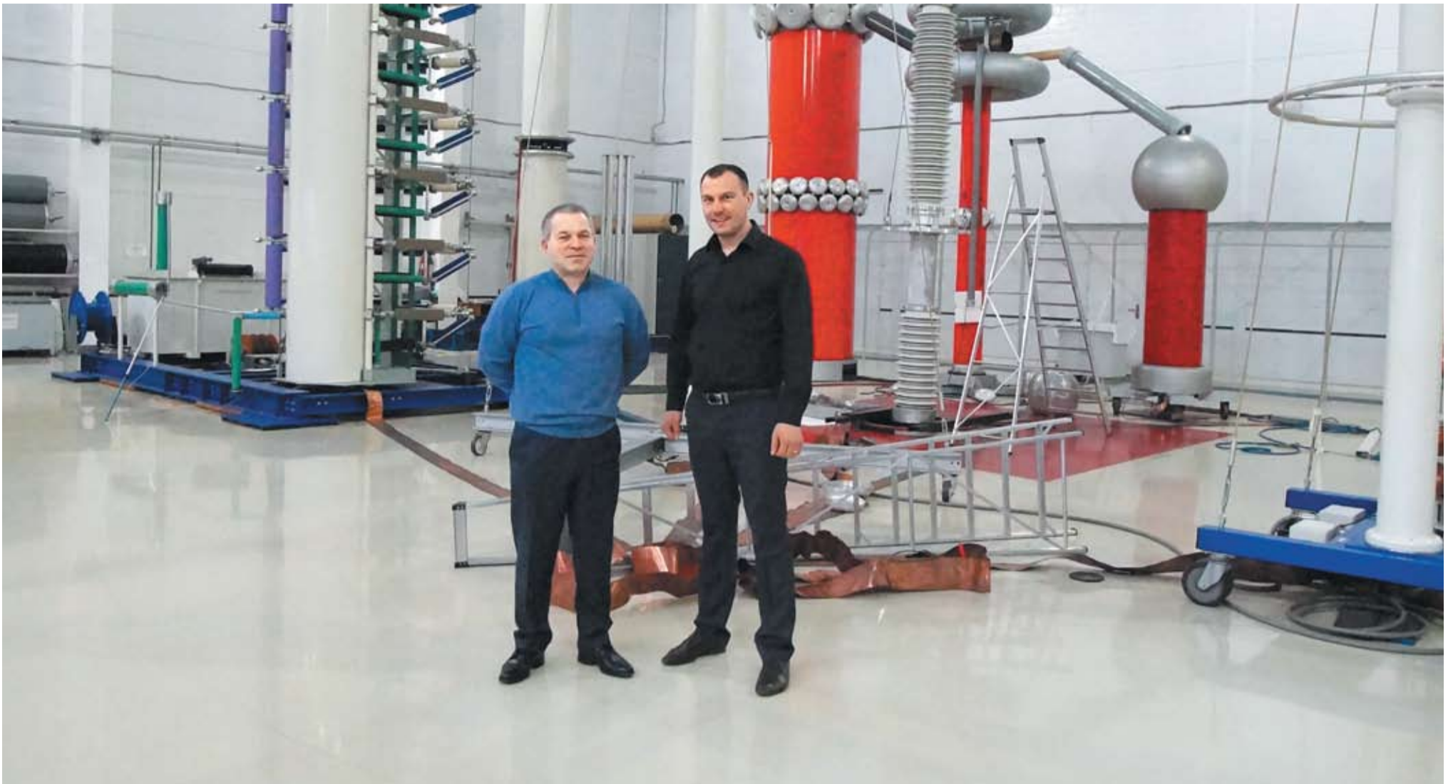
Ali Churaev (L) and Maxim Osipov at the Test Center at Izolyator plant
