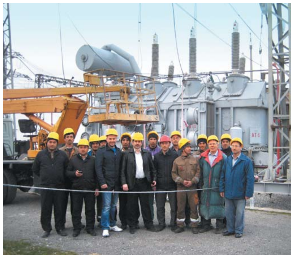
Izolyator representatives visiting Uzlovaya substation
