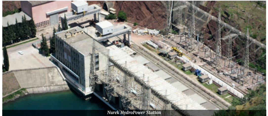
Nurek HydroPower Station
