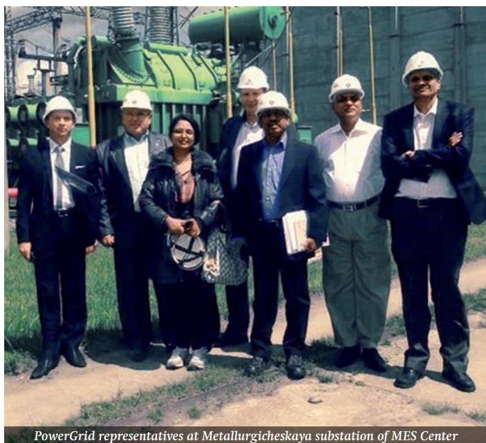
PowerGrid representatives at Metallurgicheskaya substation of MES Center
