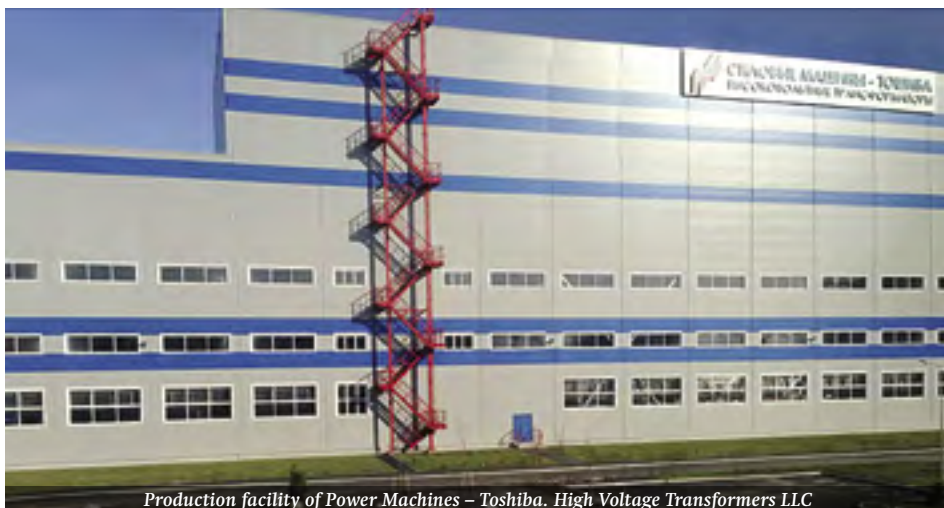
Production facility of Power Machines – Toshiba. High Voltage Transformers LLC
