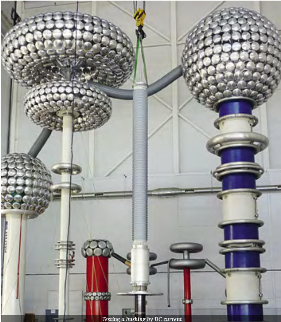
Testing a bushing by DC current
